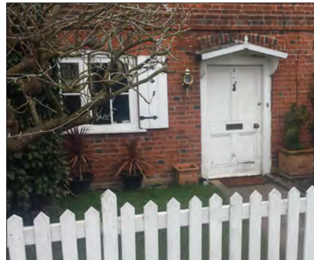
Timber windows doors and picket fence
