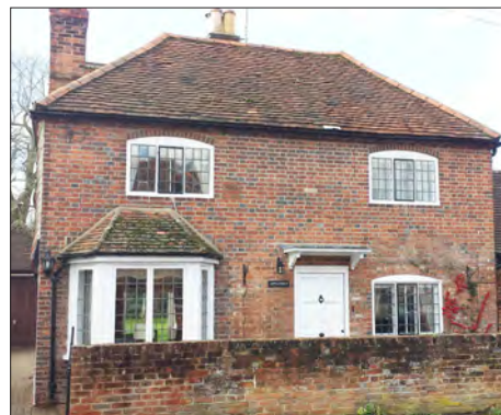
Original details all intact
