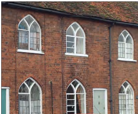
Gothic arch leaded light windows
