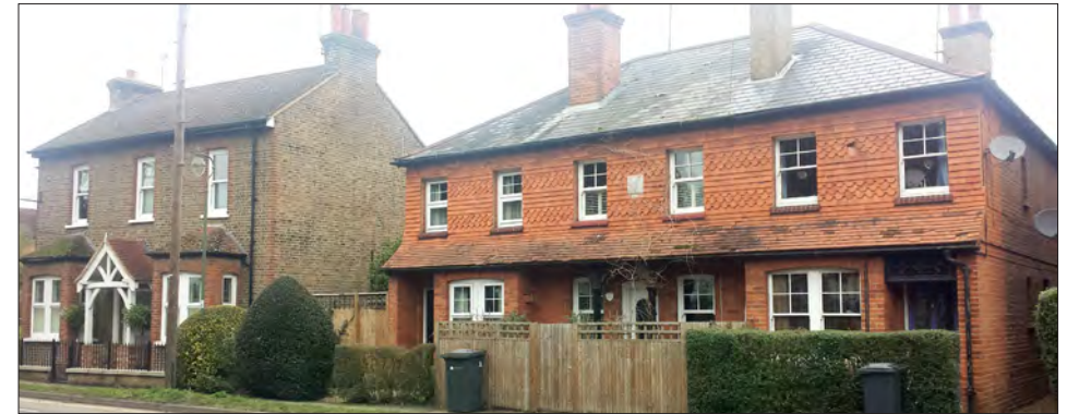
Slate roofs, brick and decorative tile hanging
