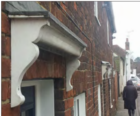
Timber door hoods
