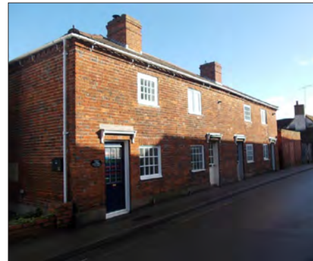
Cottages in Newark Lane
