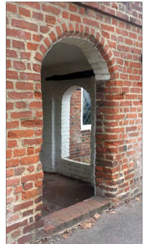
Entrance to Manor House, High Street
