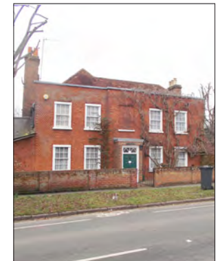
Brick re-fronting to timber frame building
