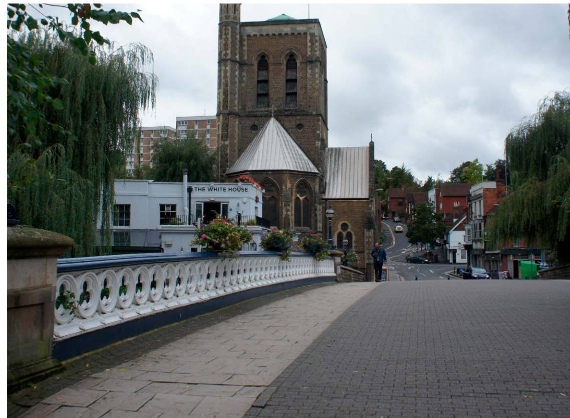
Existing photographs of the Town Bridge
