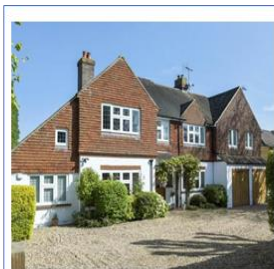
A good example of a 'wall dormer' roof, with clay tile facing and half rendered.
