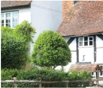
Typical timber frame/rendered building with clay tile hipped roof
