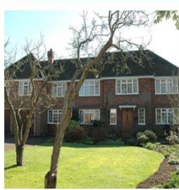
Typical example of wide, narrow property set back from the road
