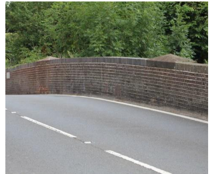
Clandon Railway Bridge
