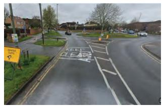
Figure 79. Example of SUP to be widened and uncontrolled crossing / pedestrian refuge to be upgraded to parallel crossing. Source: Google Street View.
