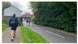
Figure 137. Uncontrolled crossing with footway missing on western side of The Street.
