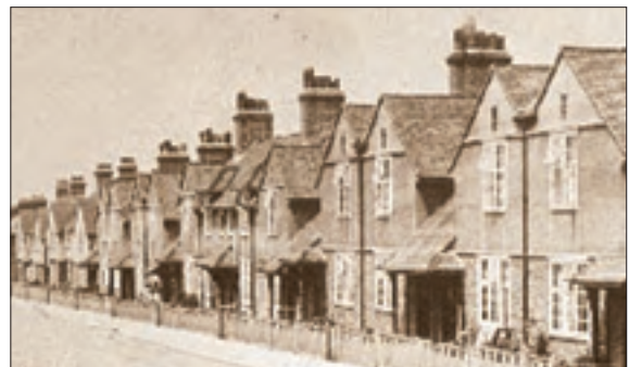
Guildford's first council houses in Cline Road, built in 1906. In 1912, a further 20 houses were added.
