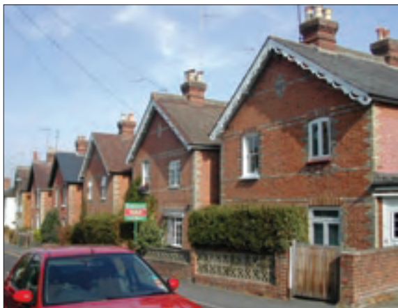
Decorative brickwork and some original door and window openings survive
