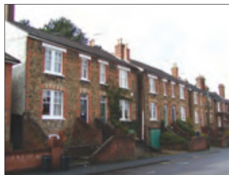
Upper floor main entrances
