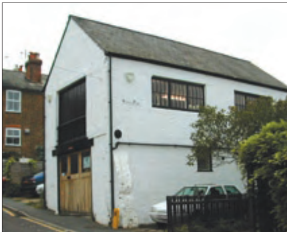
Addison Glassworks, Alexandra Place
