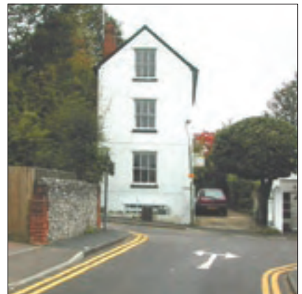
1-3 The Grove terminates the vista
