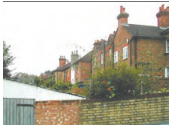
Backs of houses in Addison Road.
